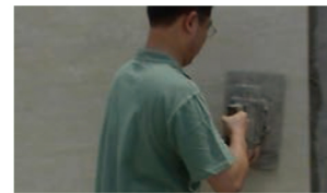
9, Press the porcelain panel by the oscillator
