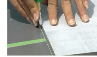
2A, Cut the porcelain panel by glass cutter
