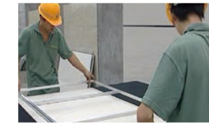
5, Join the porcelain panel with aluminum bar as a component
