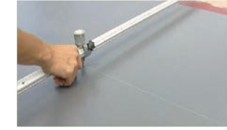
2B, Cut the porcelain panel by the push-type broach
