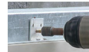
8, Screw the fabricated component on the main frame
