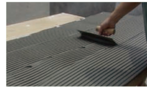
6, Use notched trowel to comb the adhesive evenly and fully onto the back of panel
