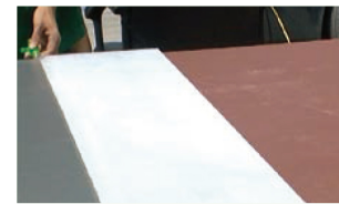
3, Put the glass cutter under the porcelain panel
