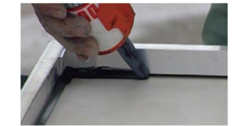
6, Fill in structural silicone sealant
