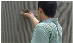
4, Use notched trowel to comb the adhesive evenly and fully onto the substrate
