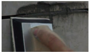
10, Fill the joint with the grout
