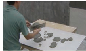
5, Apply adhesive also on the backside of the porcelain panel
