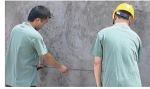
2, Draw the horizontal lines on the floor or wall, positioning with a cross line
