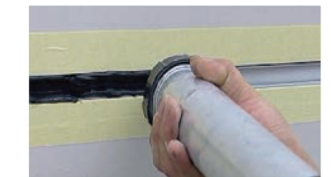
9, Fill the joint by silicone sealant
